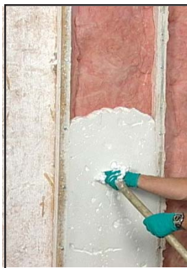
Foam flows around existing insulation in walls
