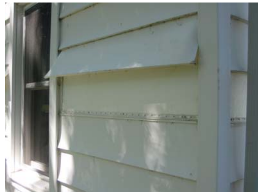
Replace Siding and Patch Holes
