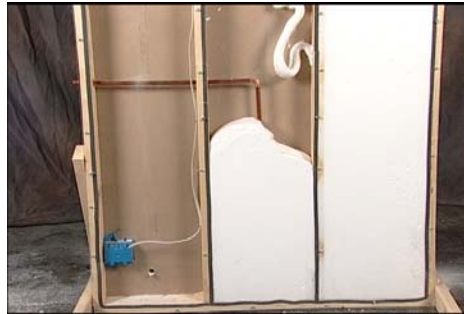
Flows around pipes, wires, and outlet boxes
