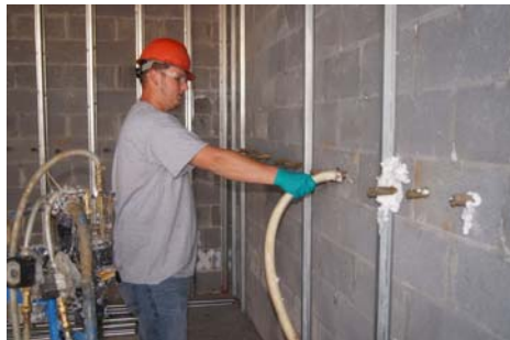
Block can be pressure injected
