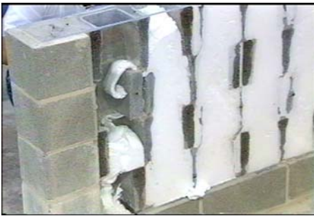
Easily flows from core to core in CMU
